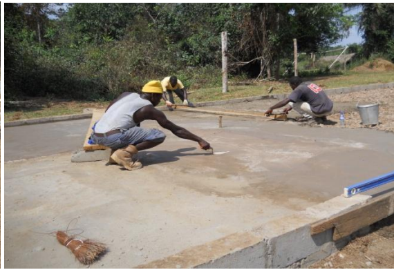
Right: Alex and Cole completing first classroom floor
