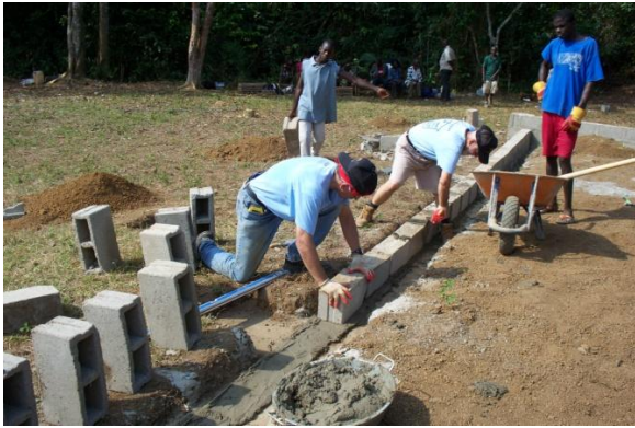
Left : George & Dennis laying concrete block walls
